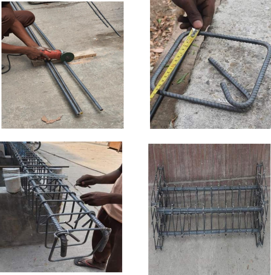
Figure 3.10: Reinforcement Preparation
