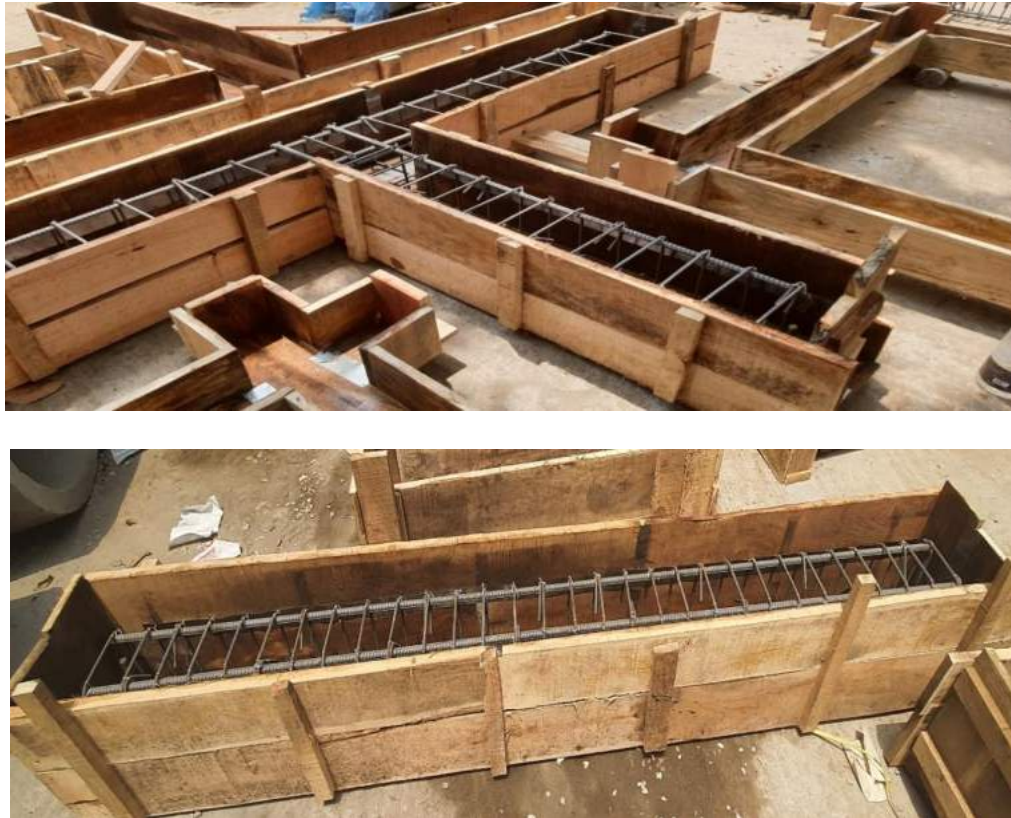
Figure 3.11: Formwork Preparation
