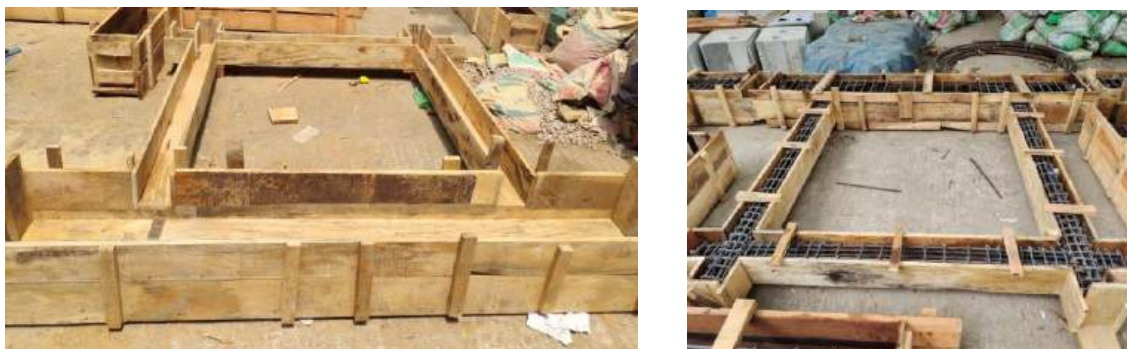
Figure 3.25- Shuttering work.
