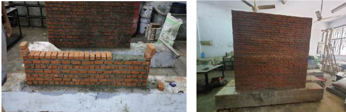
Figure 3.22- URM wall construction
