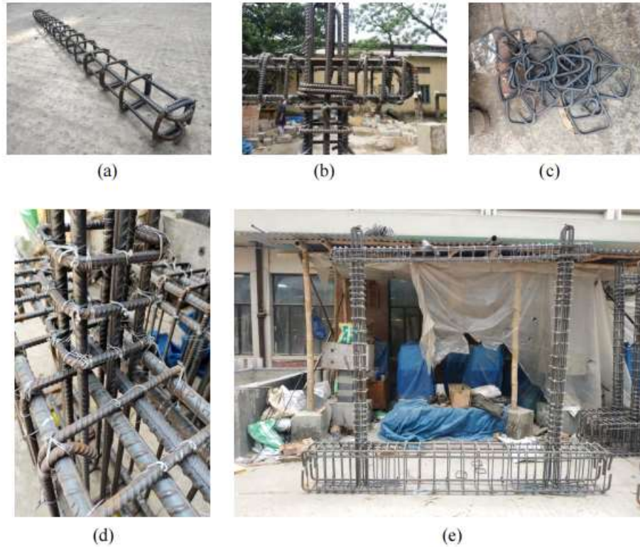
Figure 3.24- (a) lintel, (b) beam-column joint, (c) stirrups / ties, (d) column-base joint, (e) a full reinforced structure.
