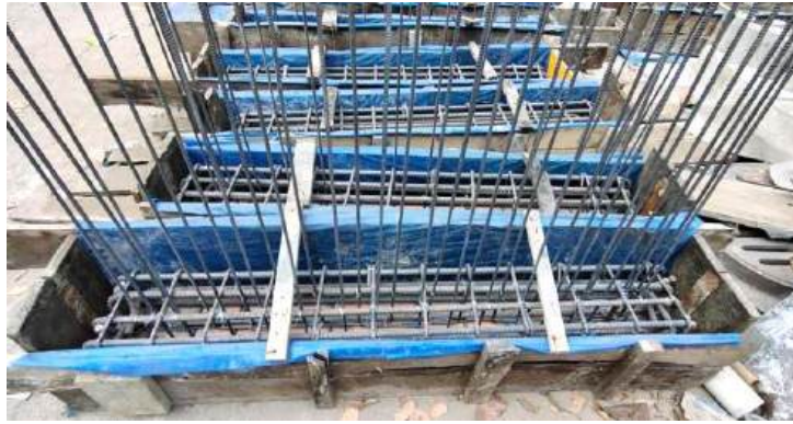
Figure 3.15- Formwork Preparation of RM walls
