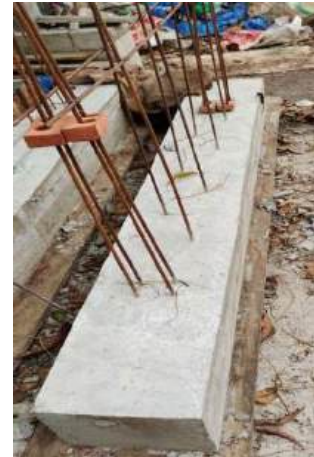
Figure 3.17- Base of RM walls after 28days of casting.
