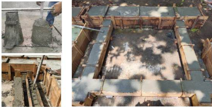
Figure 3.26- Measuring slump and concrete casting.
