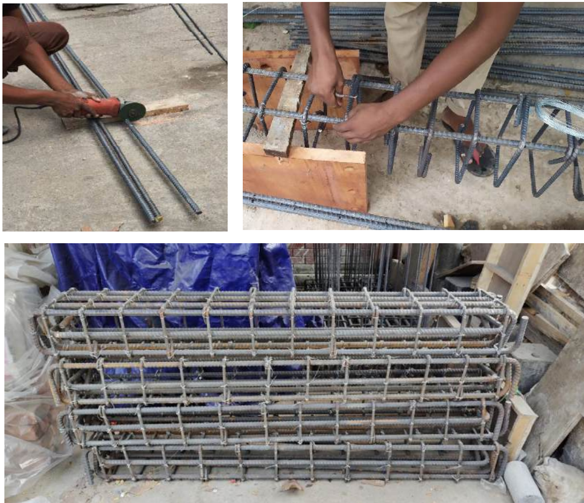
Figure 3.13- Reinforcement Preparation for base of RM walls.
