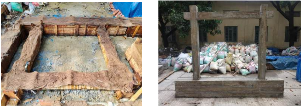
Figure 3.27- (a) curing, (b) a concrete frame after 28 days of casting.
