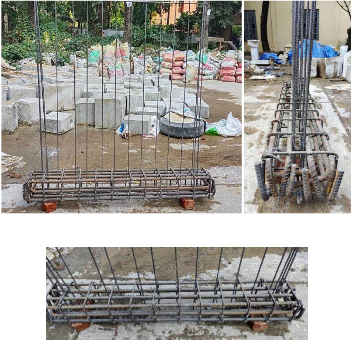
Figure 3.14- Vertical Reinforcement Preparation for base of RM
