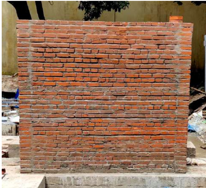
Figure 3.19- Masonry work of RM walls.
