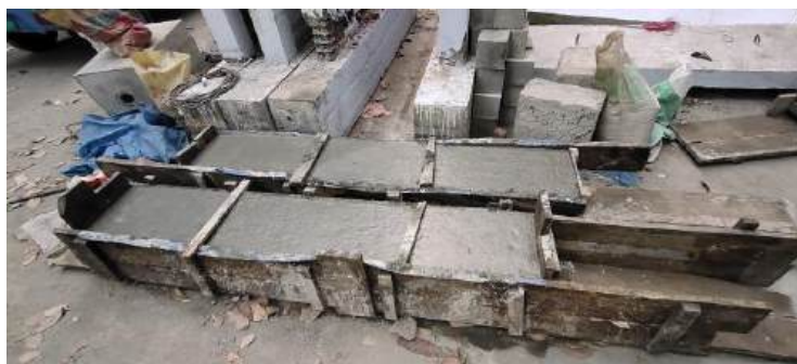
Figure 3.21- Base Construction for URM.
