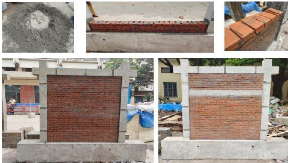
Figure 3.28- Masonry work for Infilled Frame.
