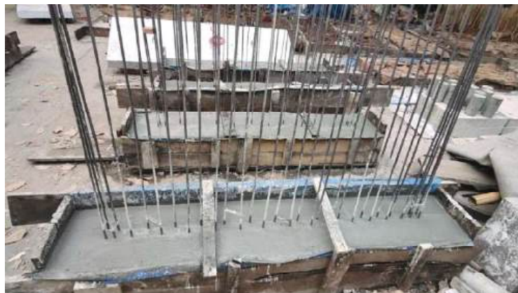
Figure 3.16- Measuring slump and concrete casting of RM walls.
